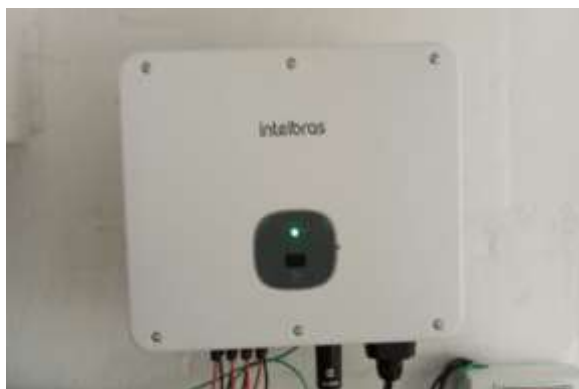
Figura 3 – Inversor On-Grid 20kW EGT 20000 MAX (380V) (Intelbras)
